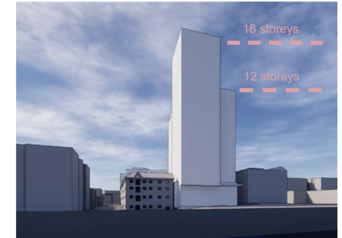
Fig. 57: View A from North side of river towards 16 storey building to Bank Place
