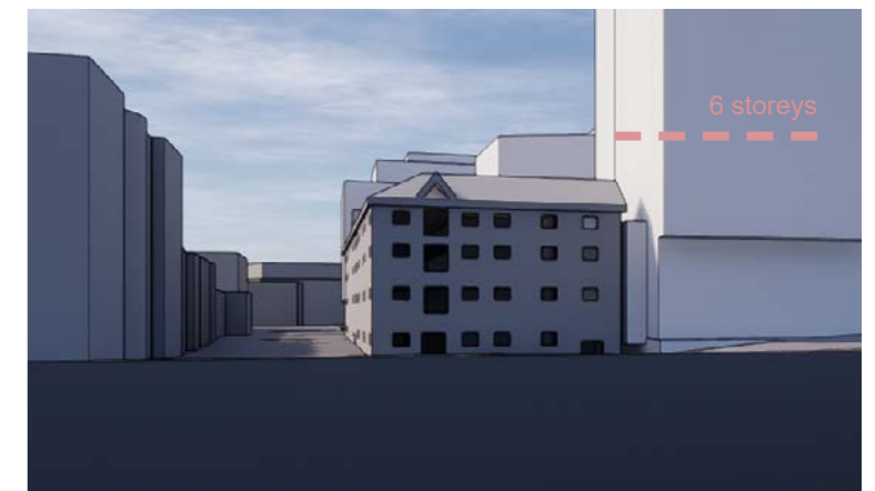
Fig. 50: View C. Granary from North with 6 storeys to new civic/commercial building within square. 6 storey element is visually evident above ridge line of the Granary Building
